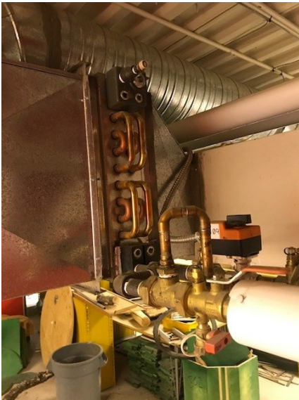
New coil and controls (Mount Sentinel)
